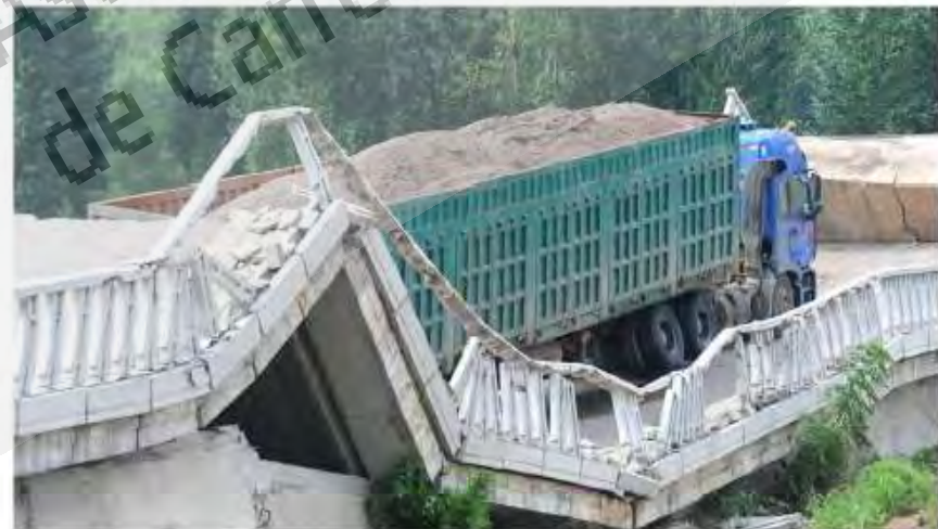
Fig. 6. Bridge collapse due to an overloaded truck (image courtesy of Yuqiang Liu)
