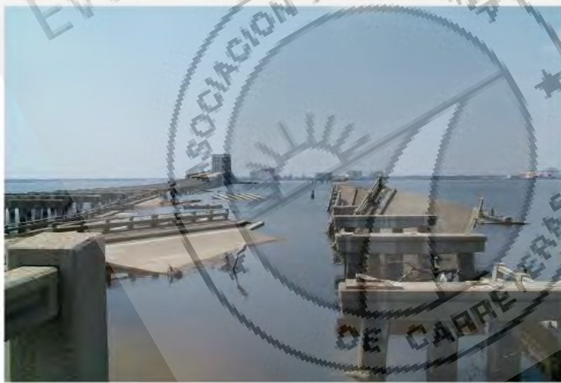
Fig. 5. Bridge decks knocked off pile caps during hurricane (image courtesy of Wikimedia Commons/Joe Furr, WIKIPEDIA 2005)
