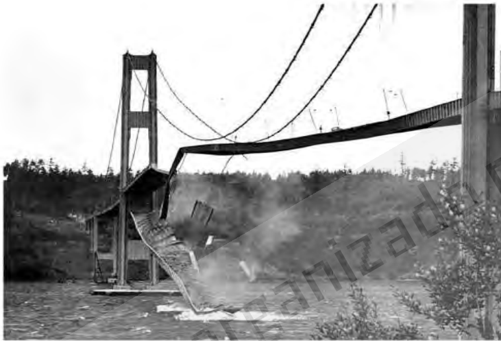
Fig. 1. Collapse of the original Tacoma Narrows Bridge in 1940 (reprinted from WIKIPEDIA 1940)
