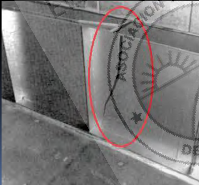
Figure 50 Fatigue Crack Through Net Section of a Tension Member
