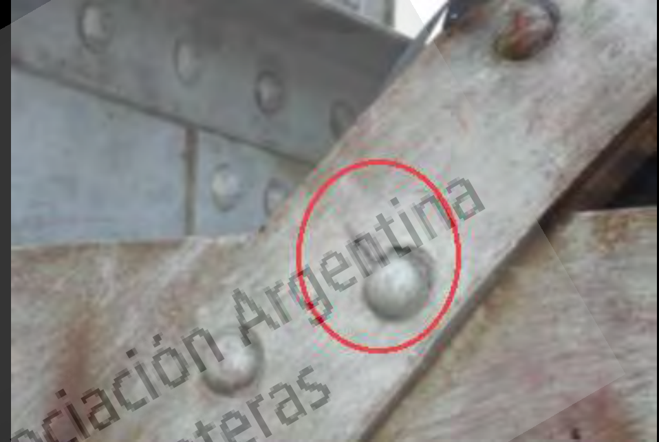
Figure 50 Fatigue Crack Through Net Section of a Tension Member
