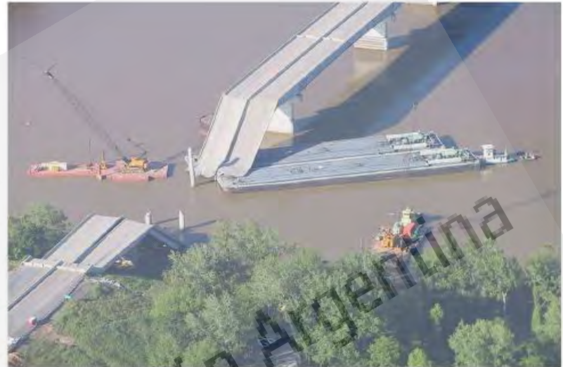
Fig. 8. Collapse of a bridge due to vessel impact (image courtesy of Wikimedia Commons/Xpda, WIKIPEDIA 2002)
