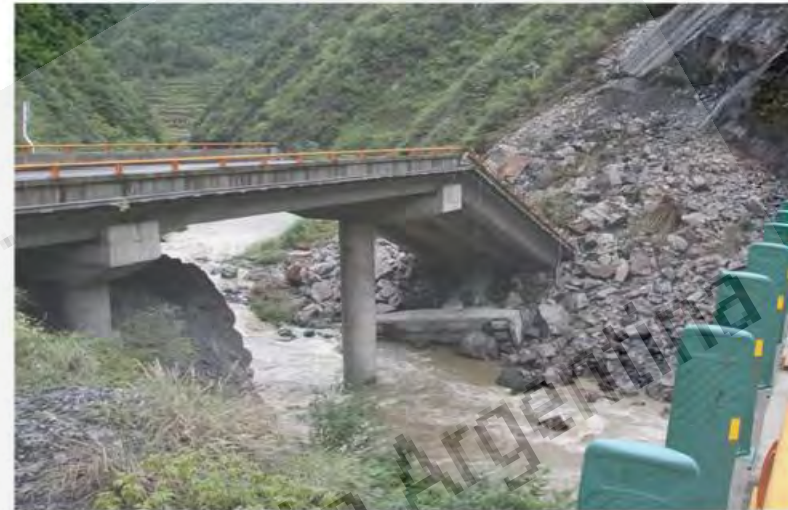
Fig. 4. Collapse of a bridge due to landslide (image courtesy of Xi Zhang)
