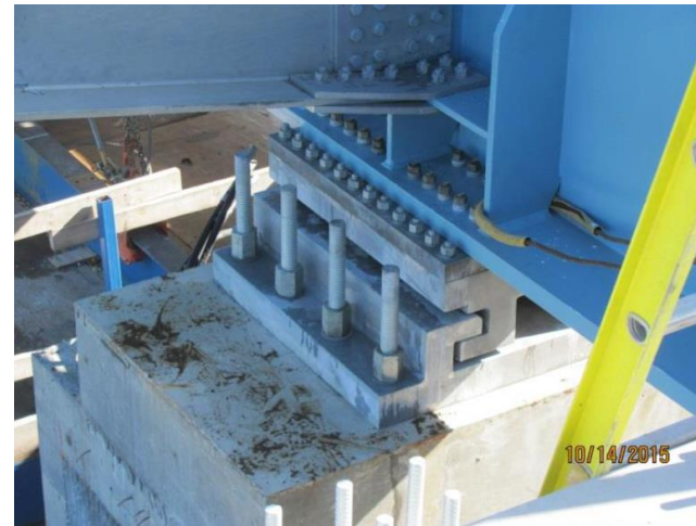
Centre-west bearing in place. Bevelled shoe plate is seen between girder flange and bearing sole plate.
