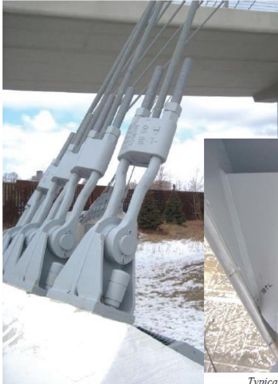
Typical cable earth anchorages.
