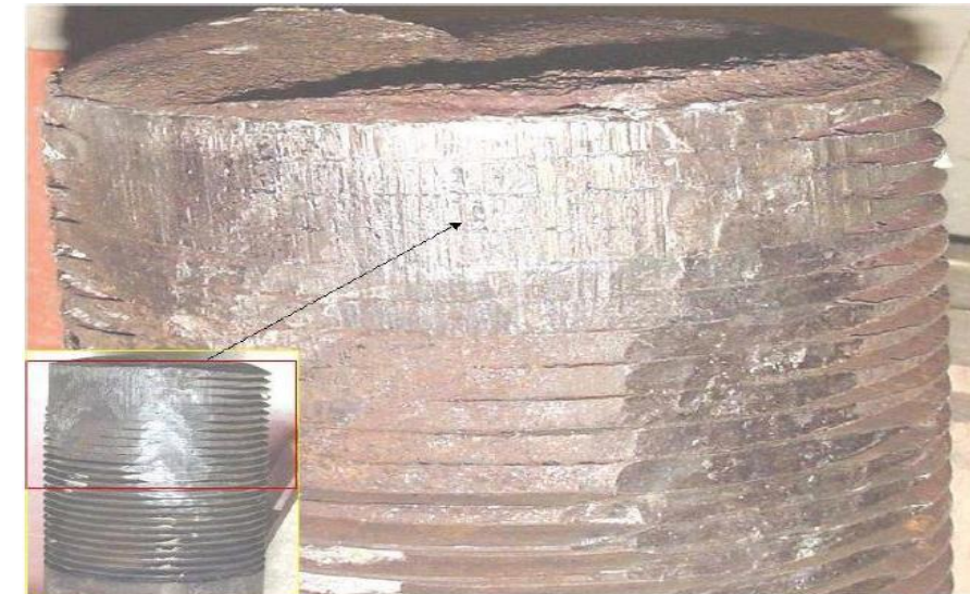
Hanger 1 (NW) – Threaded Area Showing Signs of Wear, Abrasion, and Impact Damage
