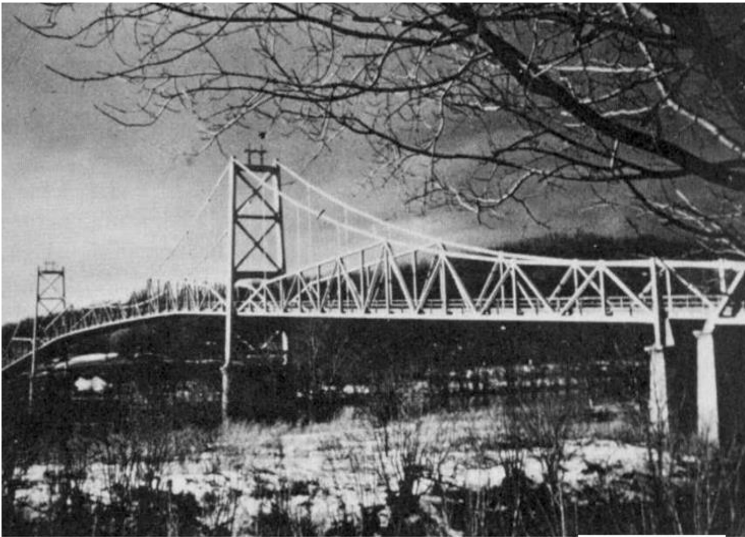
Photograph of St. Mary's bridge similar to the Pt. Pleasant bridge before collapse.
