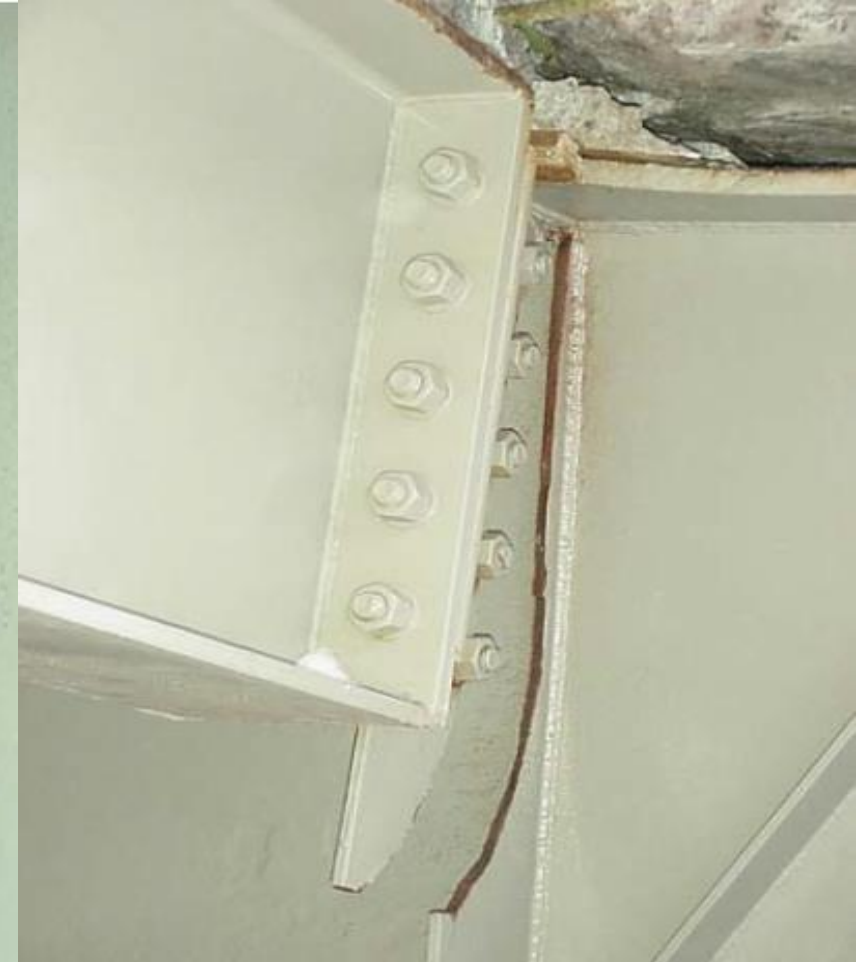
Exterior stringer to floor beam #1 connection (NW corner)
