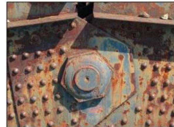
Figure 4.1.3.6 Close up Photograph of Arcola Bridge Pin Detail.
